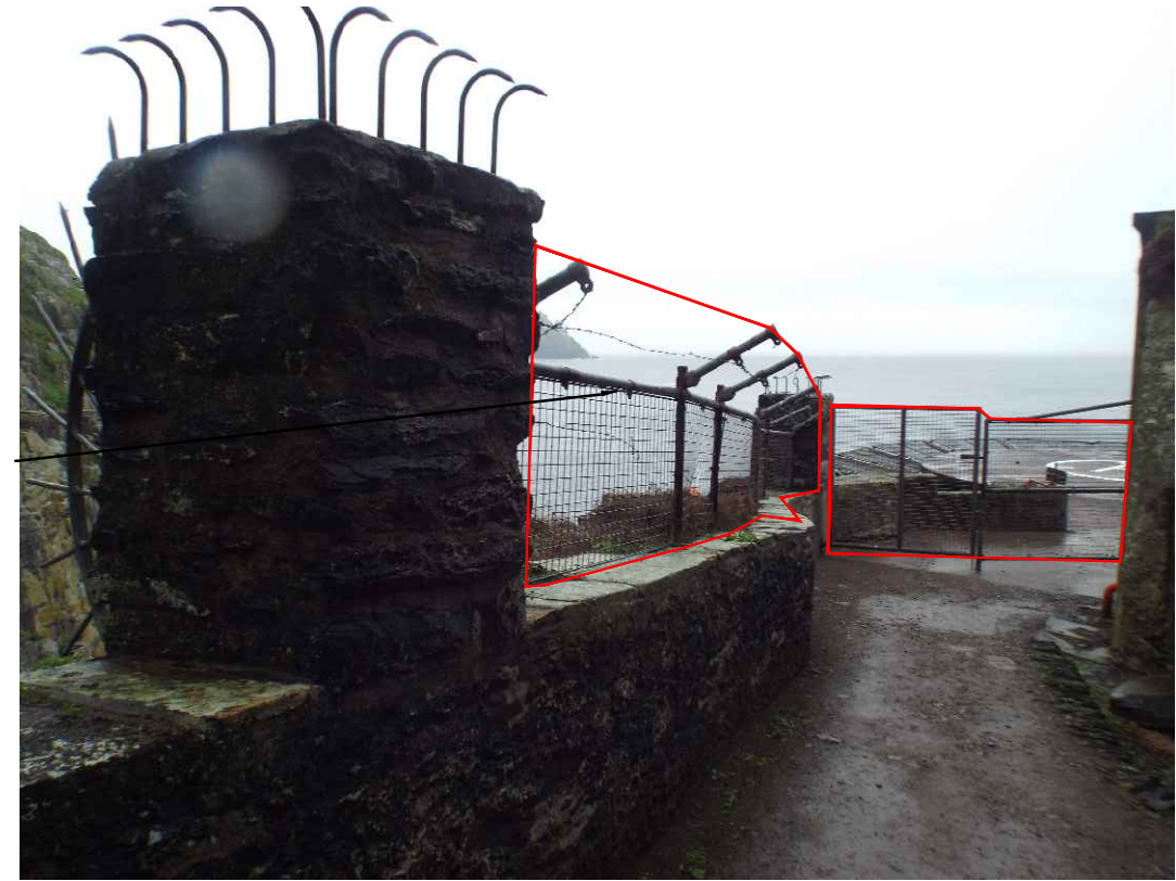
02 001 VIEW OF ENTRANCE TO HELICOPTER PAD
