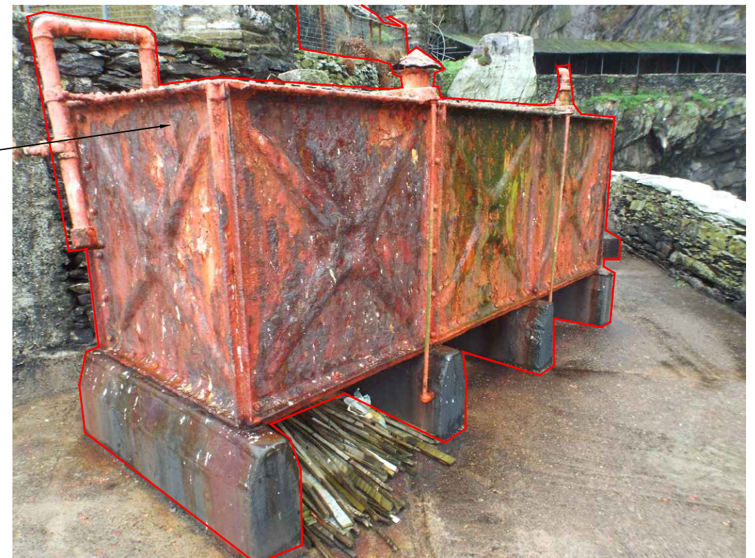
EXISTING DISUSED OIL STORAGE TANKS
