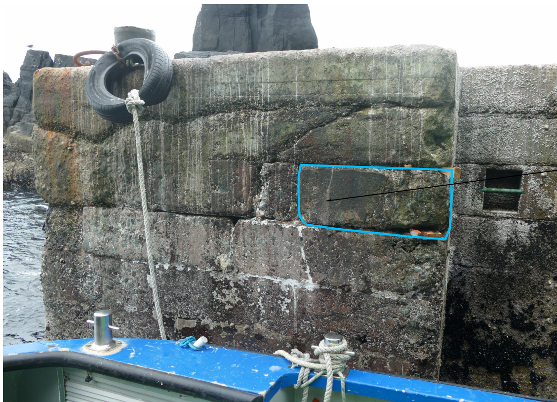
VIEW OF DAMAGE TO PIER WALL
