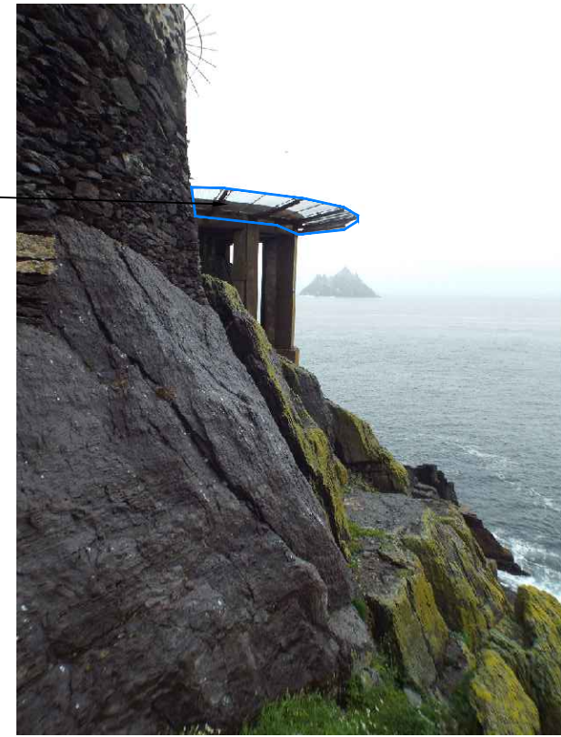
VIEW OF HELICOPTER PAD FROM BELOW
