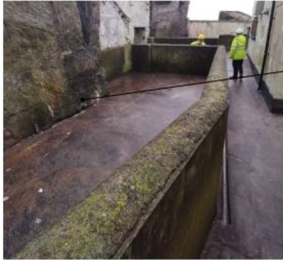
01 014 View of proposed workers toilet Location & bund walls
