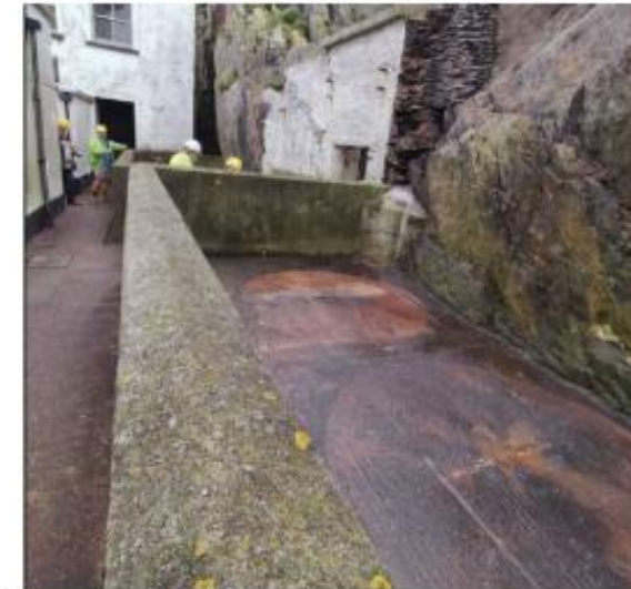
04 014 Oil tanks also removed behind second bund wall enclosure
