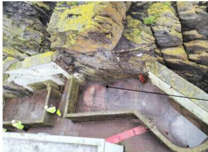
03 014 Aerial view from Lower Lighthouse Roof
