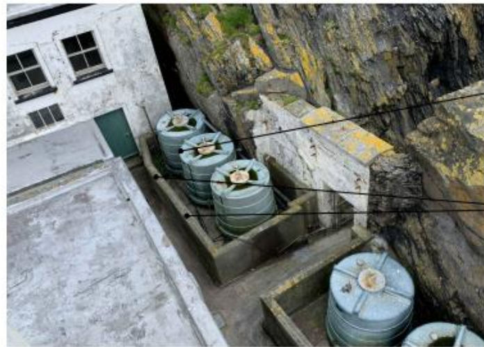
01 Existing Oil Tanks were removed during 2021 Season
