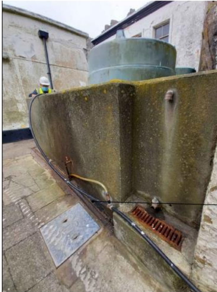
01 015 View of existing drain vent and pipework
