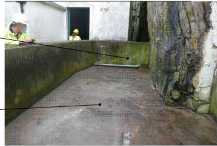
02 014 Proposed Location for workers Toilet
