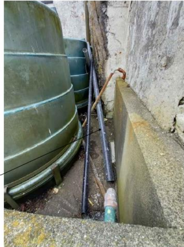
02 015 Existing pipework and Oil tanks removed during 2021 Season
