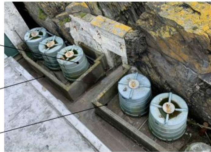
02 Existing Oil Tanks were removed during 2021 Season
