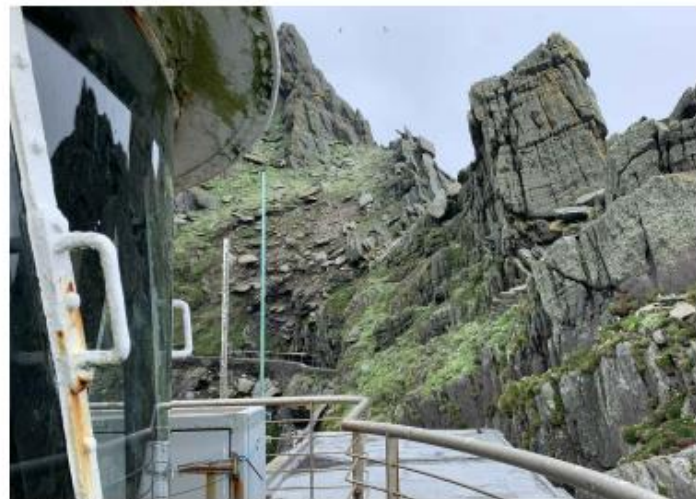
03 View from Lower Lighthouse Roof
