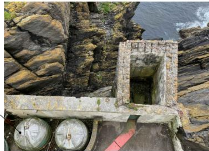
04 Existing Oil Tanks were removed during 2021 Season
