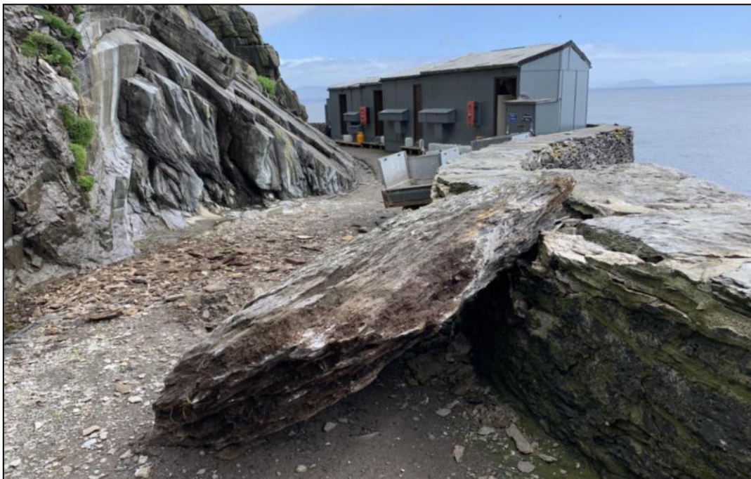
Plate 1. Displaced boulder on roadway following rock-fall near worker's accommodation huts in July 2020
