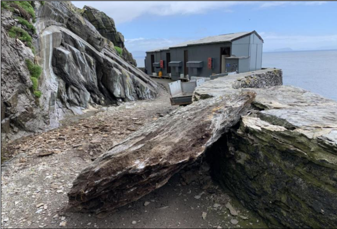
Plate 1. Displaced boulder on roadway following rock-fall near OPW accommodation huts in July 2020
