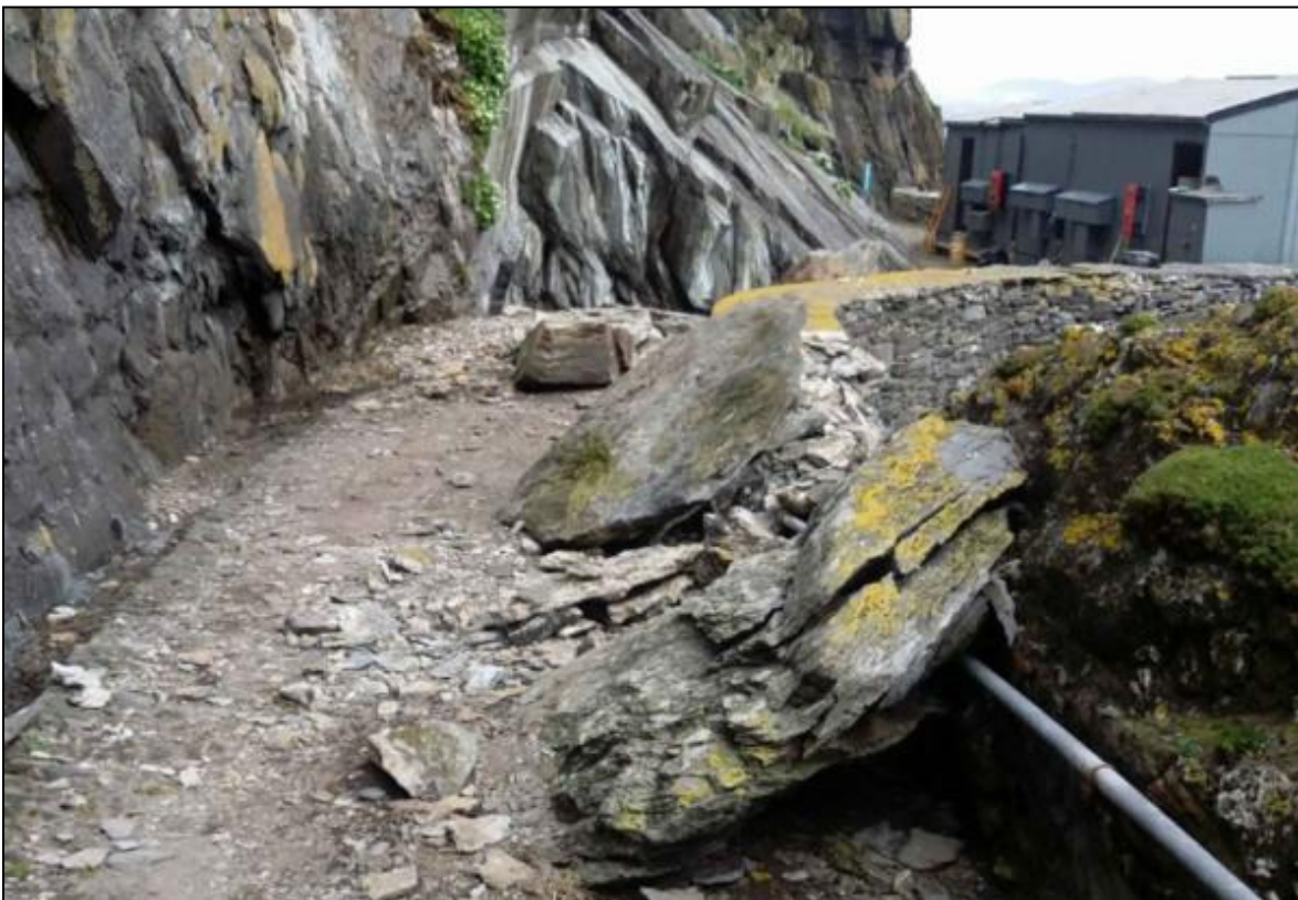
Plate 2. Displaced boulders on roadway following rock-fall near OPW accommodation huts in August 2017
