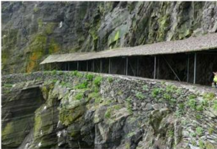
03 003 Existing crash deck at Cross Cove
