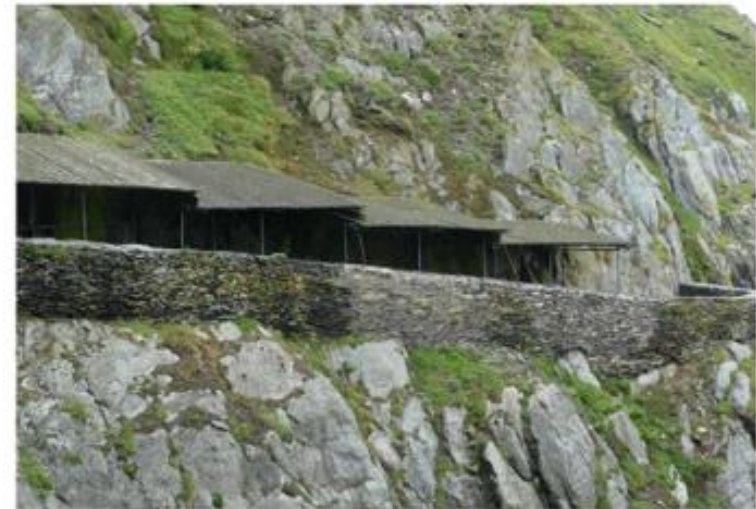
04 003 Existing crash deck at Cross Cove
