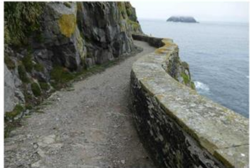
04 001 Proposed location of emergency Crash Deck on the Lower Lighthouse Road
