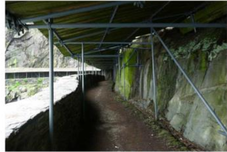
02 003 Existing crash deck at Cross Cove
