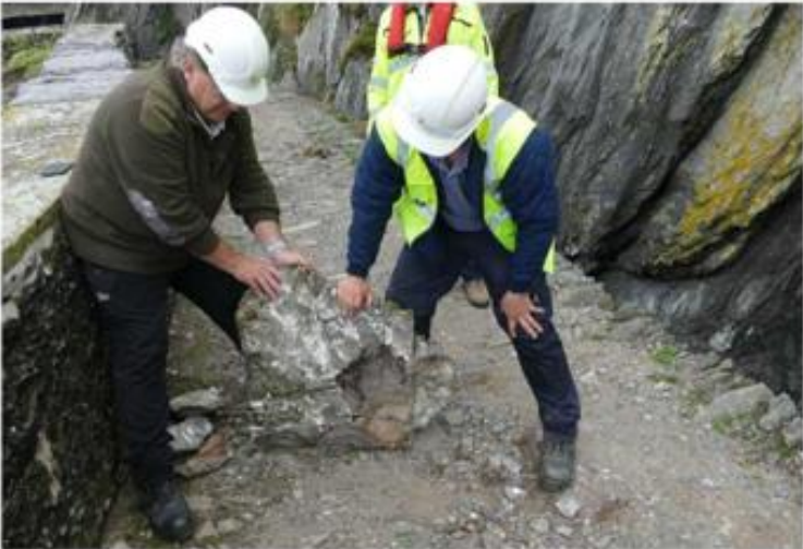
03 007 View of existing rock from the rock fall that occurred on 13.06.2022
