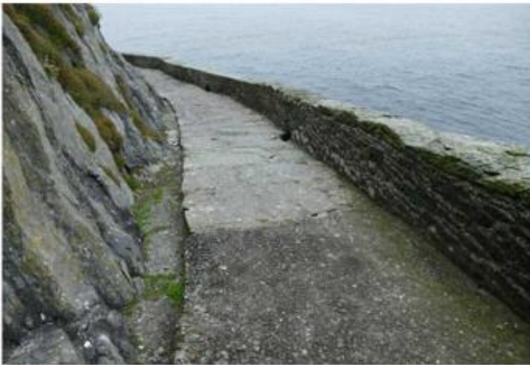
03 006 Proposed location of emergency Crash Deck on the Lower Lighthouse Road
