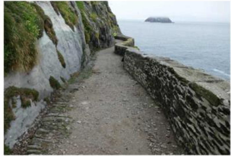
02 001 Proposed location of emergency Crash Deck on the Lower Lighthouse Road
