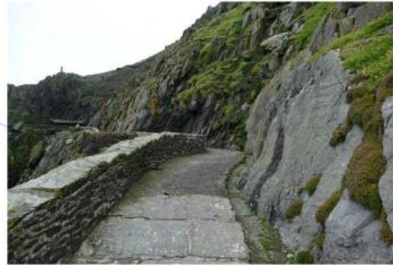
04 006 Proposed location of emergency Crash Deck on the Lower Lighthouse Road
