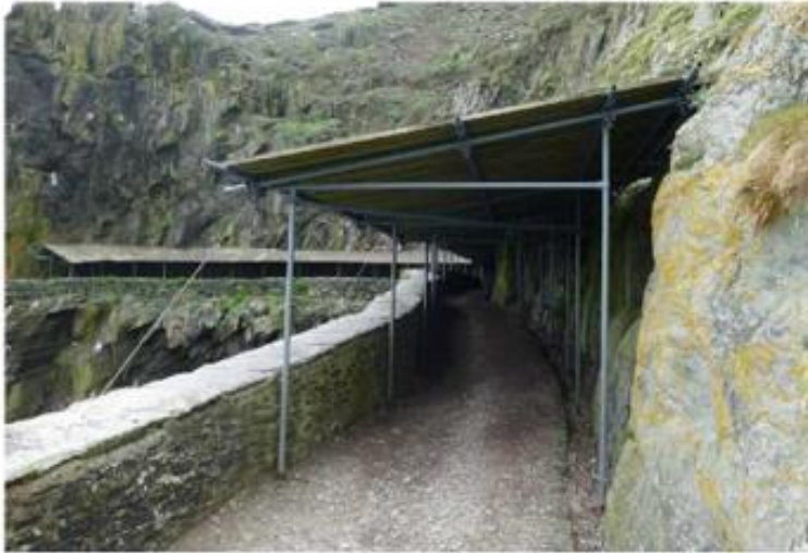
01 003 Existing crash deck at Cross Cove
