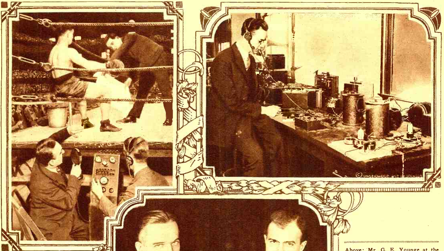
Above: Mr. G. E. Younge at the U. S. Bureau of Standards in the Act of Measuring the Frequency of a Wave Transmitted from a High Power Radio Station. The Bureau of Standards is Continually Carrying on Research Work in Radio Transmission & Reception. © Underwood & Underwood.
