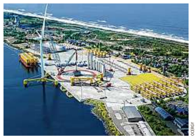
Ocergy produces offshore wind-turbine foundations.
