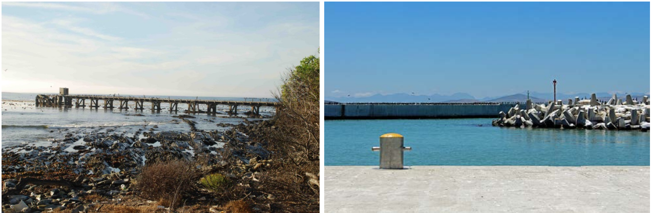
Figure 26: The old Faure Jetty (Left, photo: www.culturalheritagevalues.com ) and the new Murray's Harbour and breakwaters (right, photo: www.commonswikimedia.org ).
