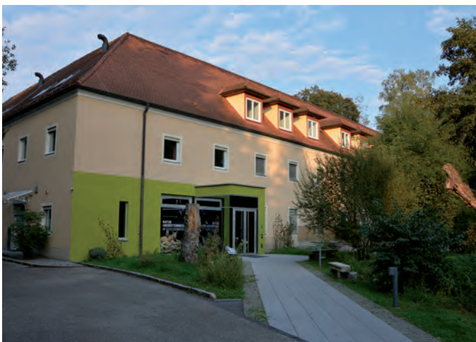
Fig. 4, 5: The Biology Centre is not a new building, but a reconstruction of the former home for the blind from 1991 till 1992. Around 155 m 2 can be used for exhibitions; guided tours are well booked. The house is surrounded by a 1,2 hectare large "Ökopark", i.e. an ecological park showing diverse biotopes including an artificial pond. Therefore, a place for teaching and recreation, which is visited by about 18,000 people per year.
