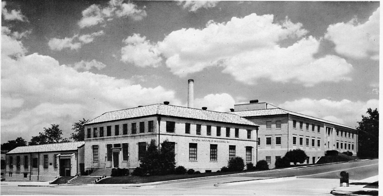
National Institute of Drycleaning: National Headquarters, Silver Spring, Maryland
