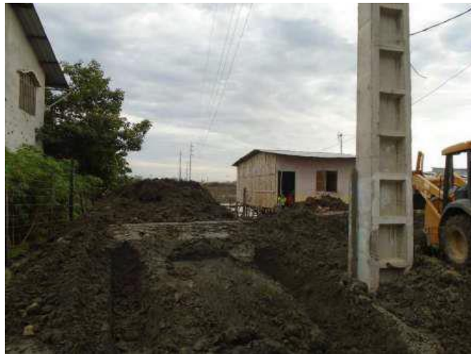
BACKFILL MATERIAL TO VIRGEN DEL CISNE SETTLEMENT
