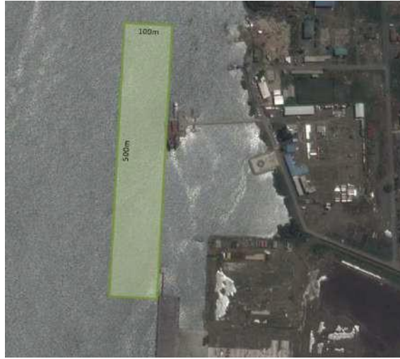
Photo 49: Dredging Area of Pier 6 DREDGING AREA PIER 6
