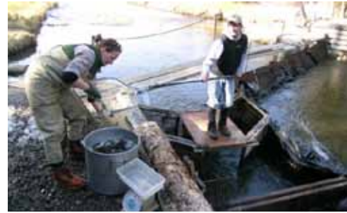
Clear Creek weir and trap rebuild. NPS Photo.
