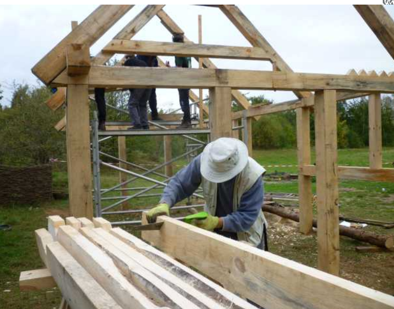
The author hard at work on a reconstruction Anglo-Saxon building, preparing rafters by sawing notches
