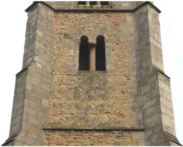
Close up of Anglo-Saxon belfry windows, showing herringbone work and coursed rubble in the walling
