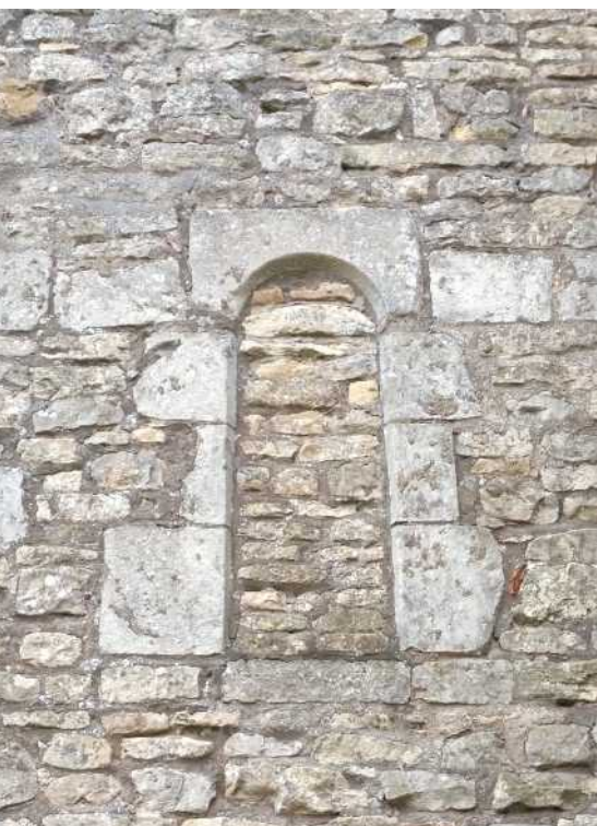
Blocked Anglo-Saxon window in the outside north wall of the chancel
