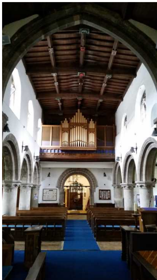
Nave looking west to tower arch. On right (north) side, the line of the scar where the Anglo-Saxon walls stop and the 15th century ones start can be seen cutting through the clerestory windows
